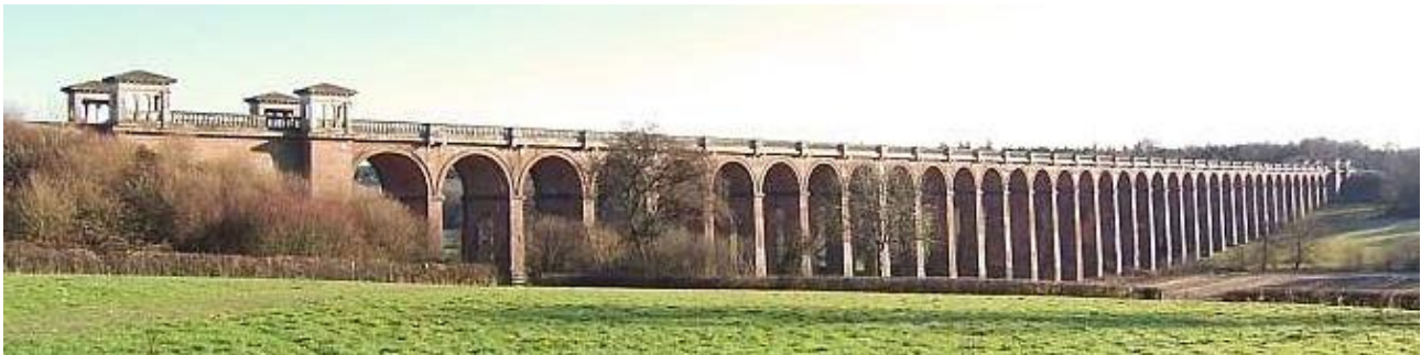
Figure 1: Ouse valley viaduct
