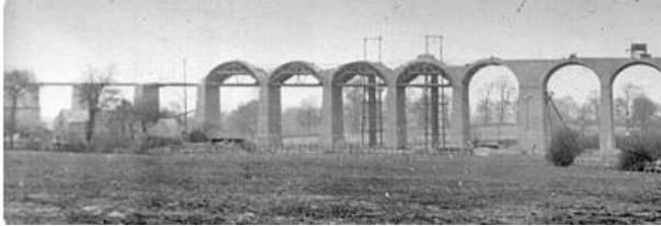
Figure 10: Sequential arch construction
