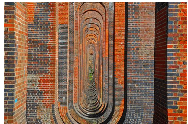
Figure 5: Opposing brickwork within piers
