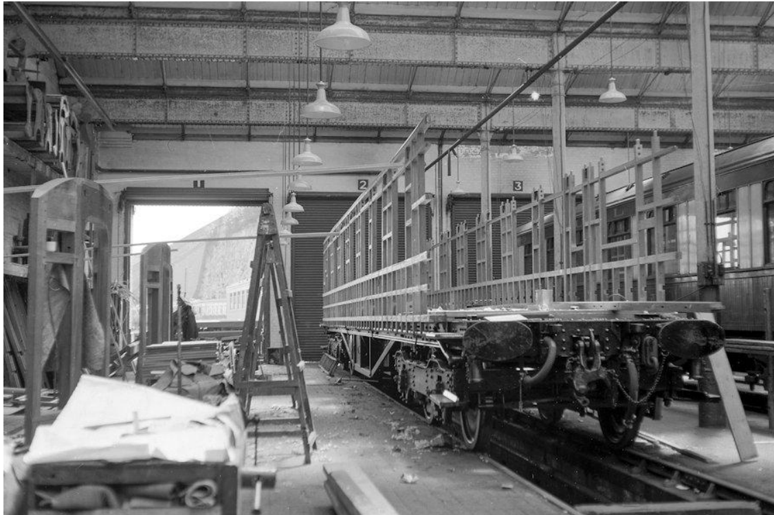
CW014-26 - May 30 th , 1951 - Pullman 1st Class Kitchen Car 'ARIES' under construction at Preston Park Pullman Car Works - © Joe Kent / Bluebell Railway Museum SR Archive [091373].
