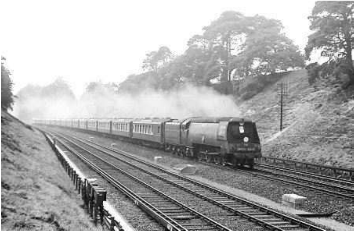
Photograph – The Mike Morant collection
