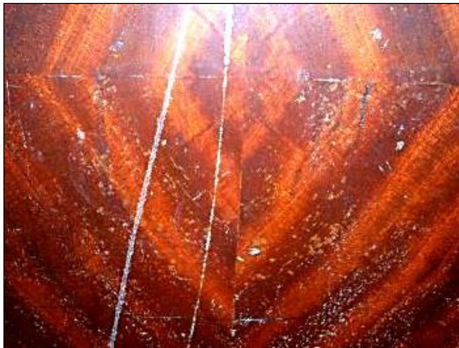
A close view of the damage sustained in over 60 years of storage.
