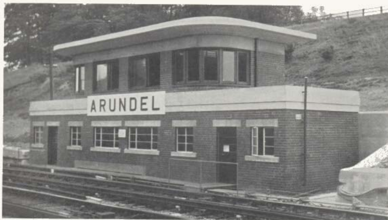
The new electro-mechanically equipped box at Arundel
