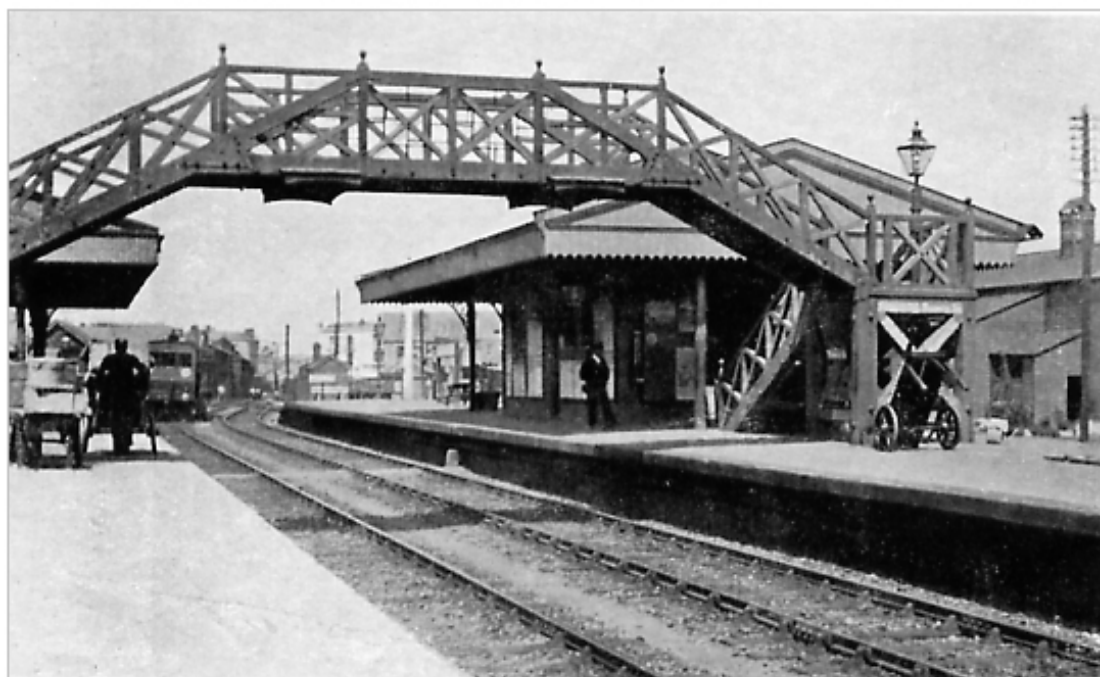
Wadebridge Station, looking towards Padstow, in L.S.W.R. days. Rail motor at down platform
