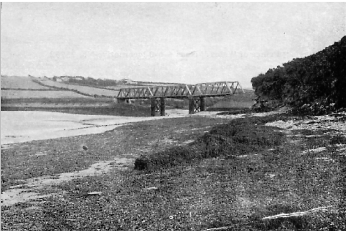
Viaduct over creek at Little Petherick, near Padstow
