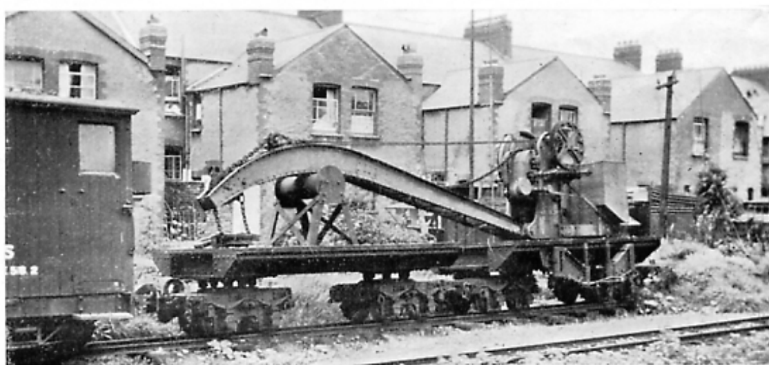
Crane at Pilton
