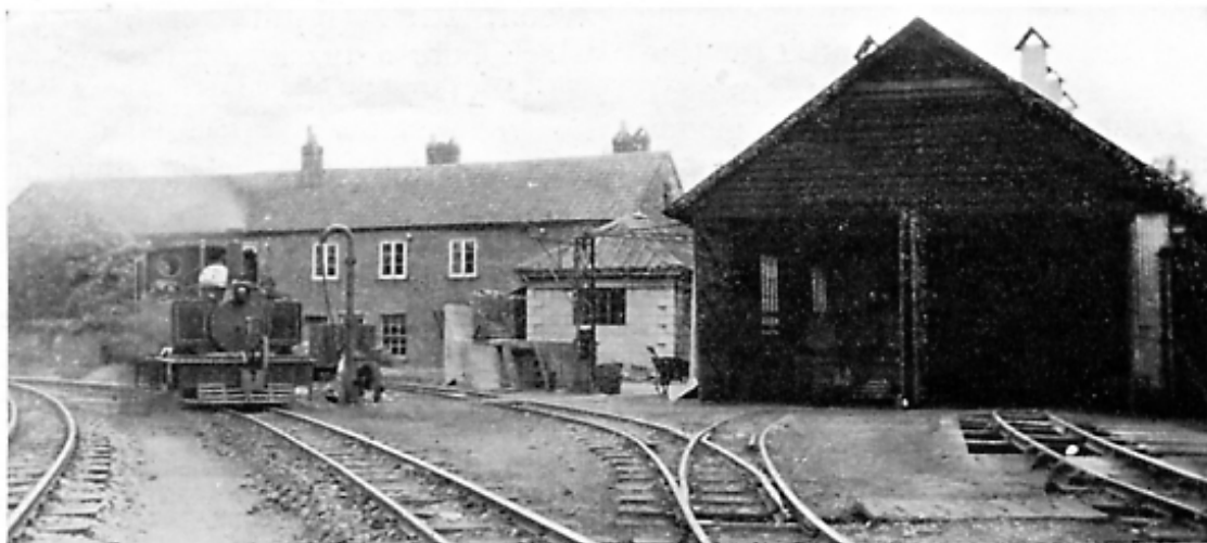
The old general offices of the Lynton & Barnstaple Railway, with existing engine shed at Pilton yard
