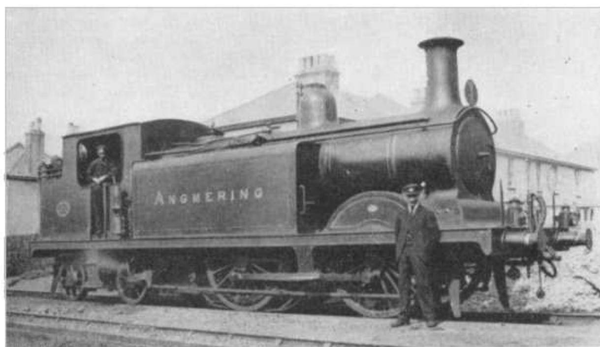
L.B.S.C.R. "D3" class 0-4-4 tank engine No. 371, "Angmering," as originally built, at Littlehampton in 1901
