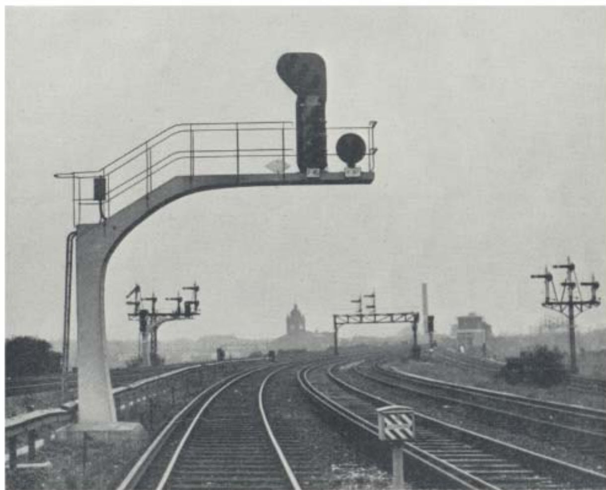
Bricklayers Arms Junction down spur inner home signal. Colour-light signals have now replaced the semaphore arms in the background
