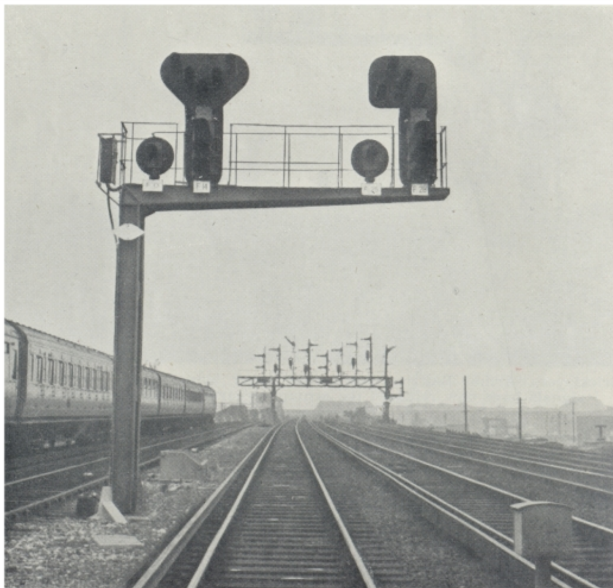
Bricklayers Arms Junction up through and local home signals, showing the up home signals and approach lights of the former signalling system in the background
