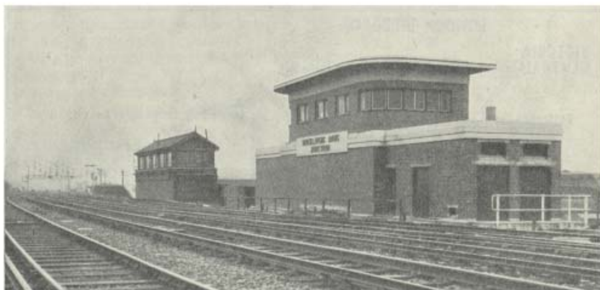
The new all-electric signalbox at Bricklayers Arms Junction. The existing signal box, on the left, is to be demolished
