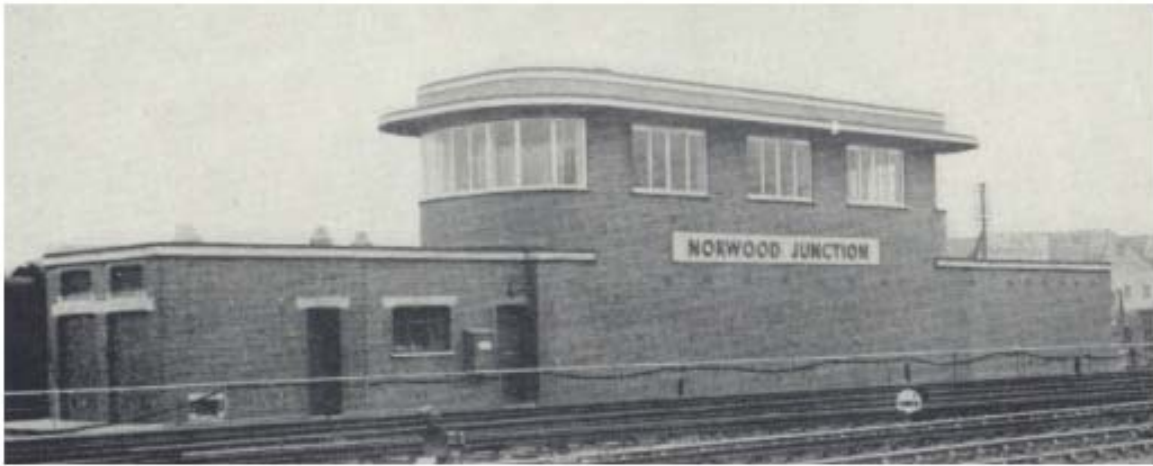
The new all-electric signalbox at Norwood Junction, which has replaced two manually-operated boxes
