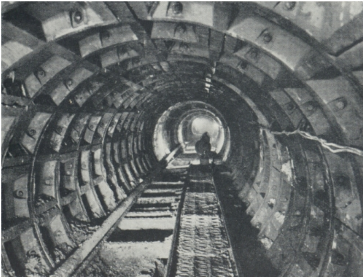
The new 6 ft. 6 in. drainage tunnel driven into the cliff
