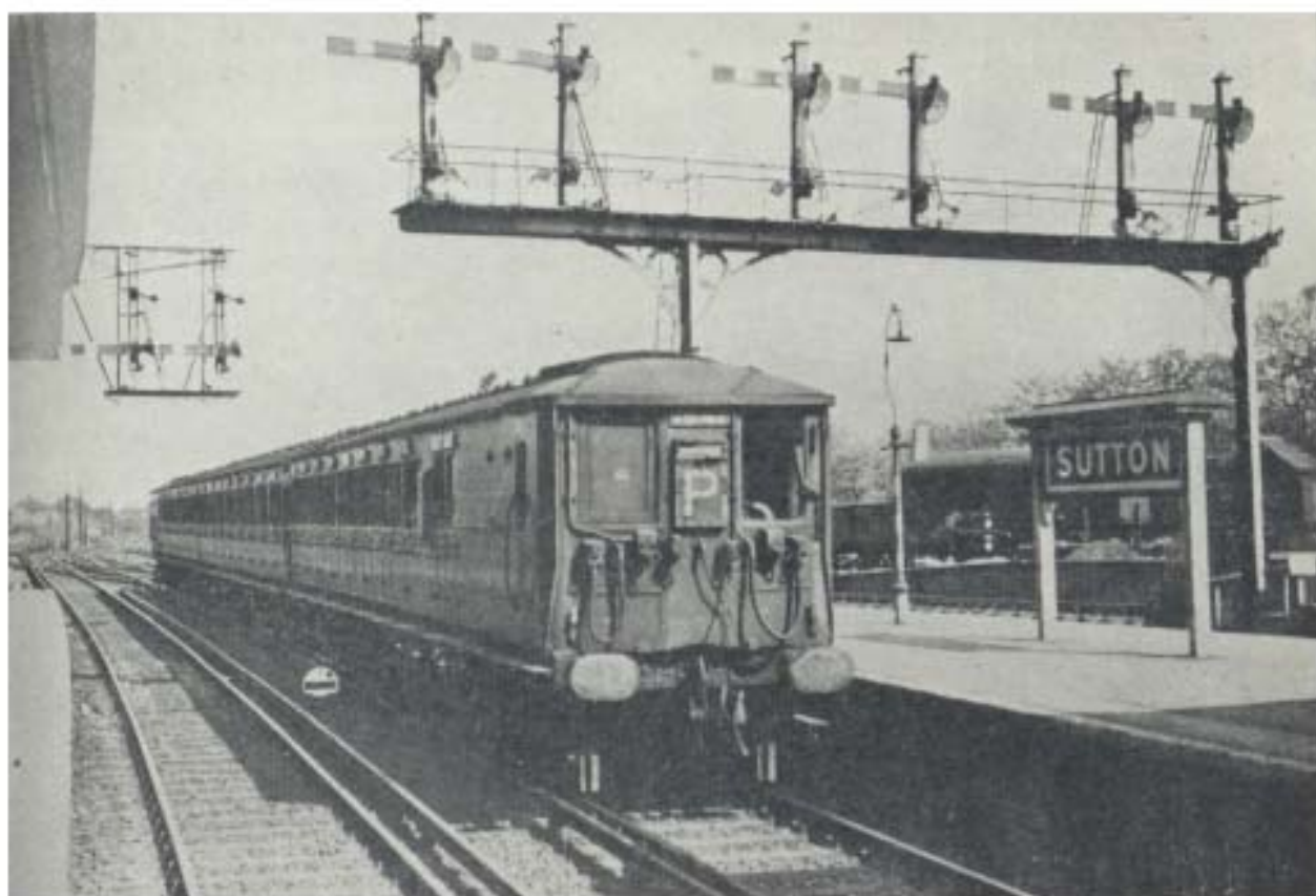
West Croydon-Holborn Viaduct train entering Sutton
