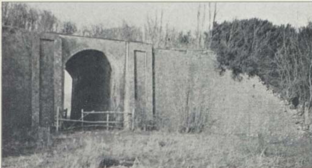
An abandoned underbridge and embankment near Uckfield
